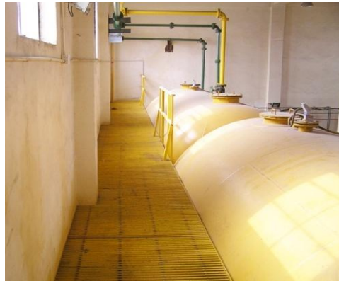
Industrial platform and walkways
